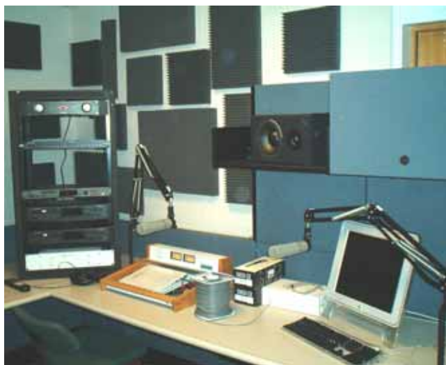
KFSR's new production facility takes shape
